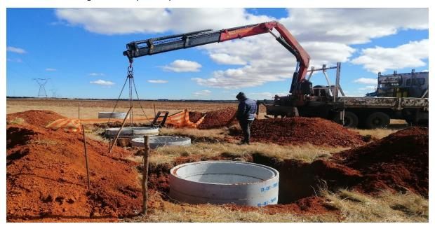
Figure 3: Fitting of concrete rings into excavations.
